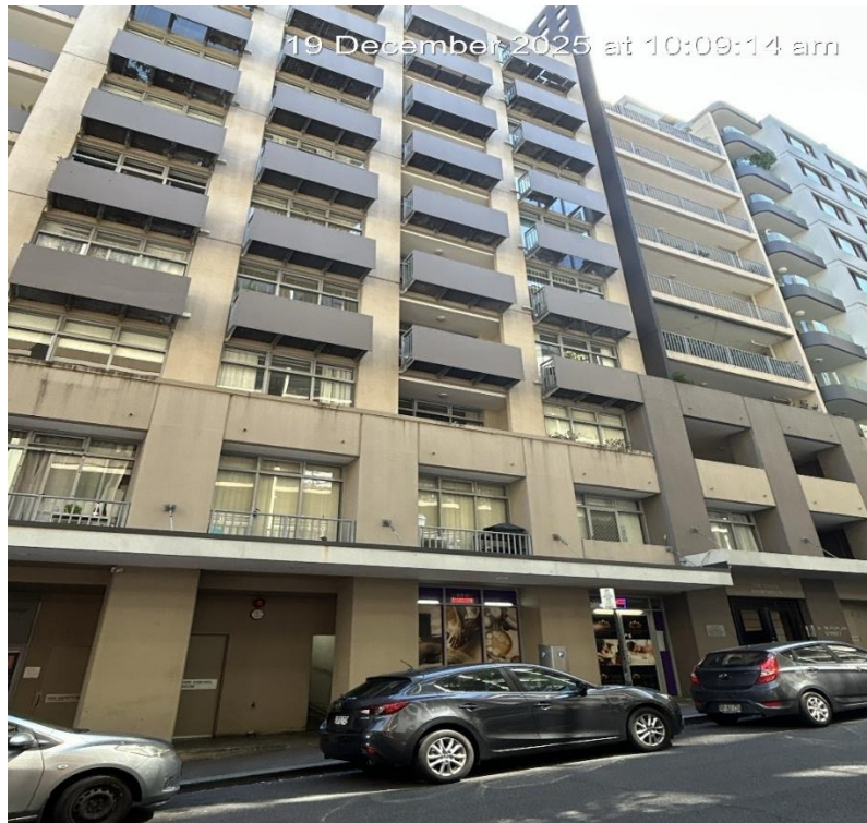
Figure 1: 6-18 Poplar Street, Surry Hills, viewed from the north
